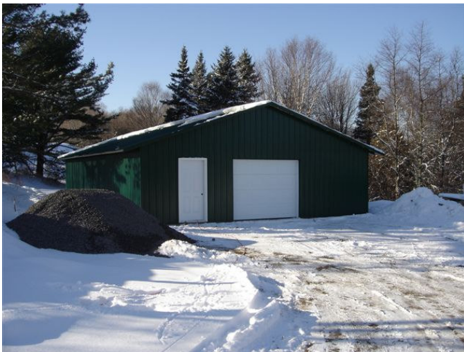
Westfield's New Power Cart Storage Shed
